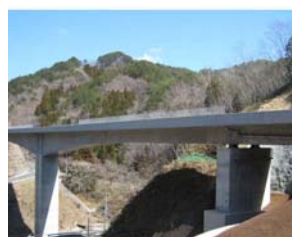
Fig-1 Ryoishi Viaduct
