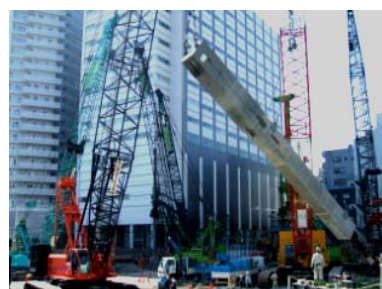
Erection of HSPC basement column
