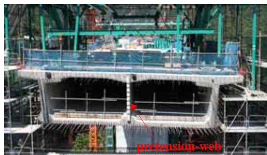
Fig-1 General view of girder section
