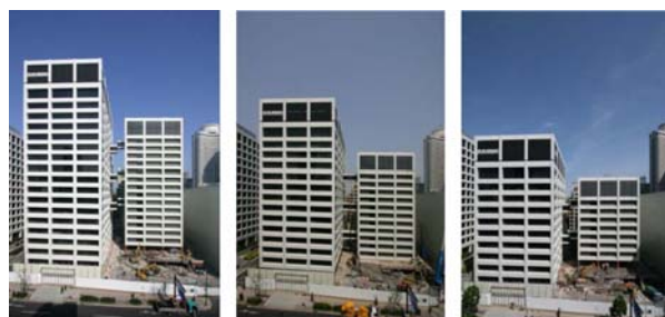
Demolition progress (March · April · May 2008)
