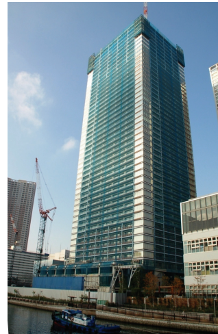
Photo 1 Appearance under construction
