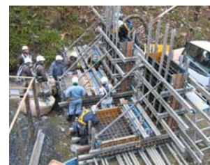
Fig-3 Pumping test
