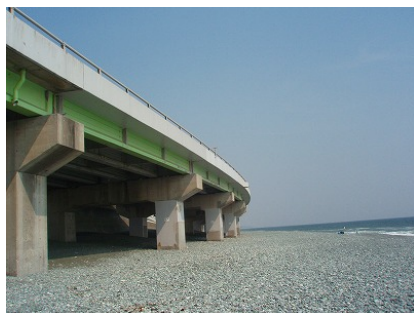
Phot.1 Sourou Bridge
