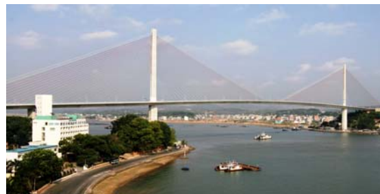
Fig.1 Bai Chay Bridge
