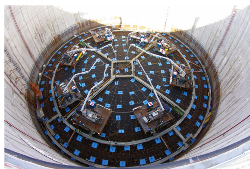
Photo1 View of Concrete Work of Bottom Slab
