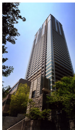
Photo-1 Complete view
