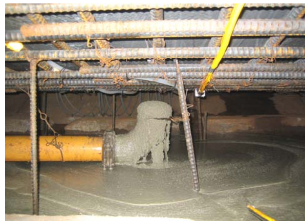
Photo 1 Placement of the concrete for the bottom lift.
