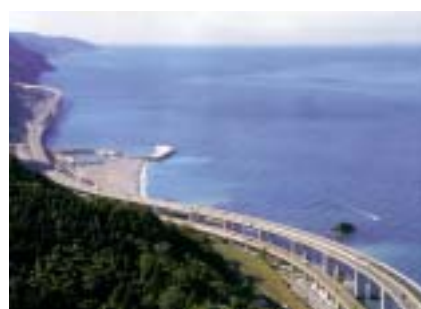
Fig.1 Oyashirazu Seaside Bridge
