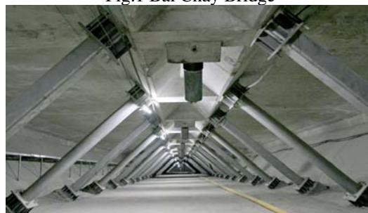
Fig.2 Steel Pipe Bracing
