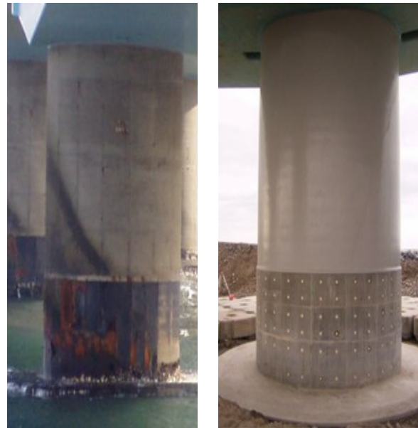
Photo 1 Pier before and after work
