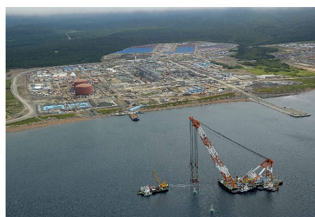
Photo.1 LNG plant and oil export terminal
