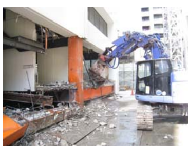
Demolition work at the ground.
