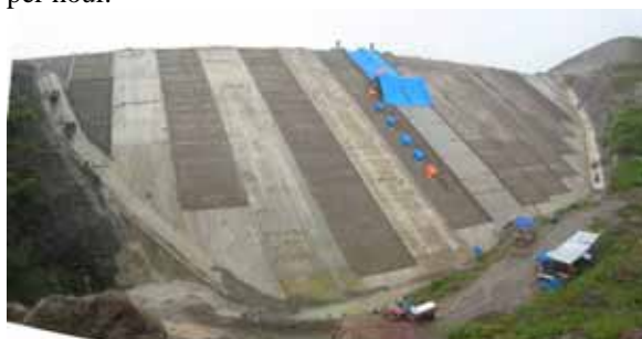
Photo 1 Concrete Face Slab by Using a Slipform
