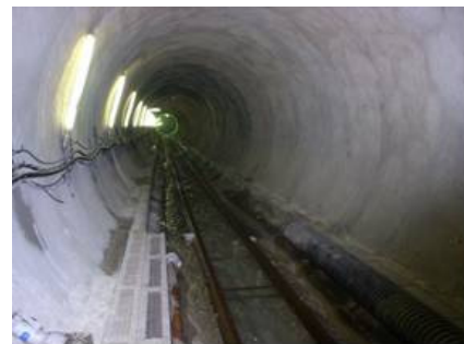
Photo.2 Completion Situation of Secondary Lining
