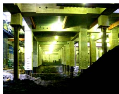
Bottom floor after excavation
