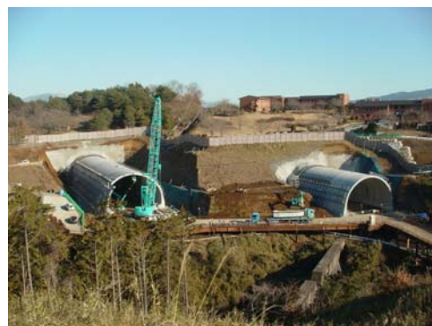
Fig.2. View of the western tunnel entrance
