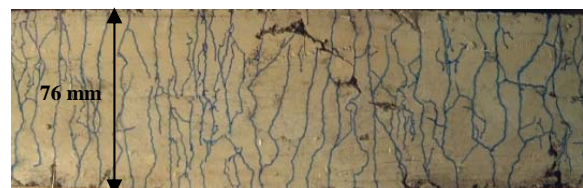
Fig.13 Crack distributions in HF-SHFRC long prismatic reinforced tensile test
