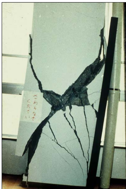
Photo 3. Shear failure
