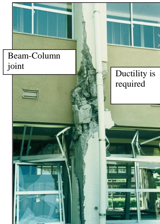
Photo 2. Beam-column joint failure
