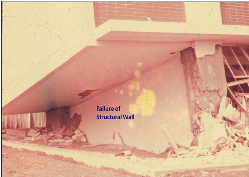
Photo 5. Failure of structural wall
