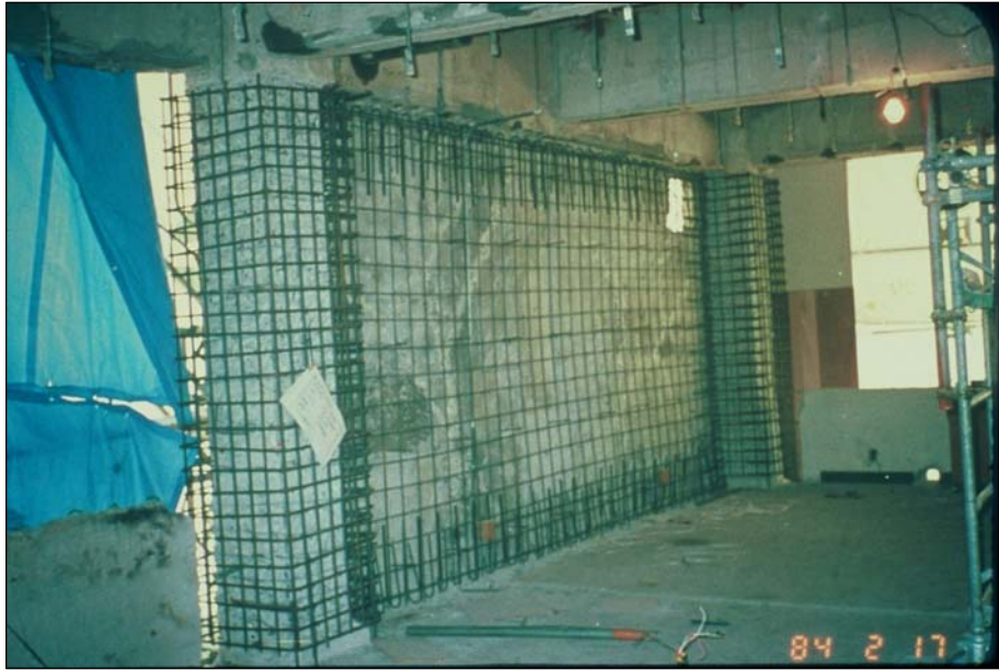
Photo 7. Increasing strength by adding a structural wall
