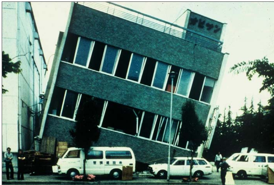
Photo 1. Unbalanced stiffness in plan
