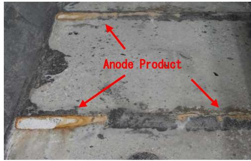
**Fig. 4: Anode product generated on line**
