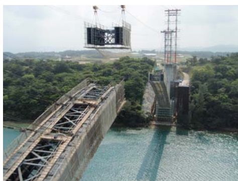
Photo.1 Construction of Warumi Bridge
