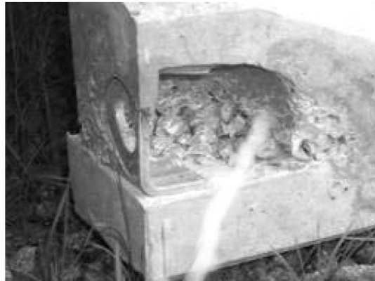
Figure 2: Example of defect (Insufficient filling at connection fitting)
