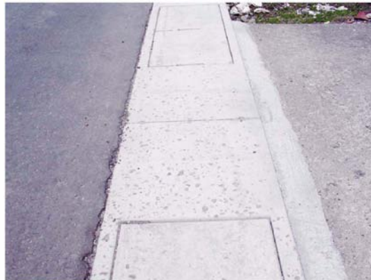
Figure 3: Example of defect (Popout due to deicing salt)
