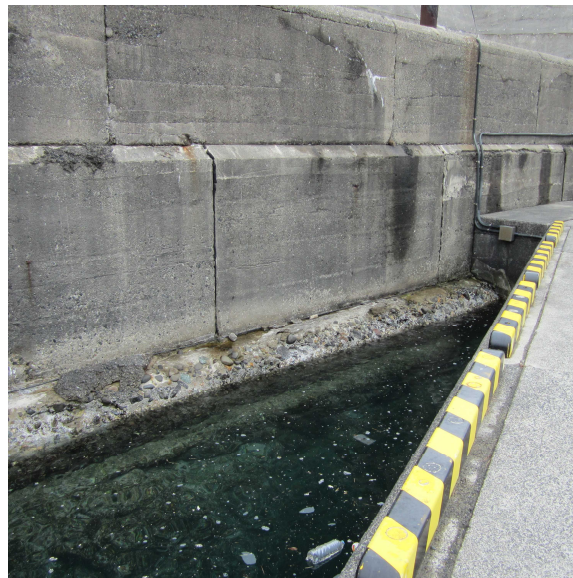
Fig. 2: Tajiri port (Tottori prefecture) -Pre-packed Concrete structure mixed with seawater-
