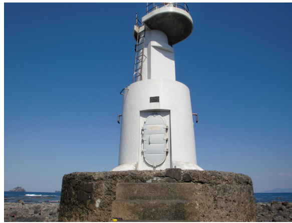
Fig. 1: Ukushima lighthouse (Nagasaki prefecture) -Concrete structure mixed with seawater-
