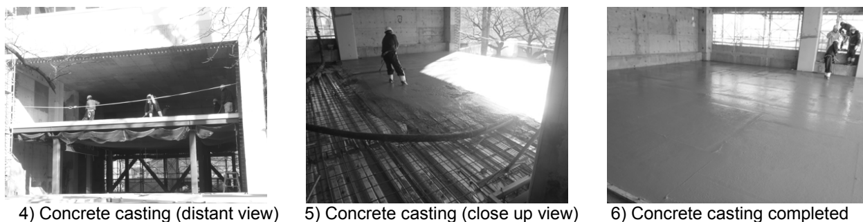
Fig. 8: Experiment on IC tag insertion into concrete at expansion floor slabs construction
