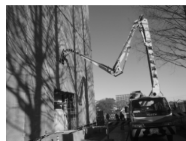
3) Pumping concrete
