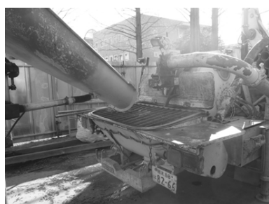
1) Pouring concrete to pumping truck
