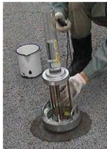
Photo-1 Example of in-situ water permeability test
