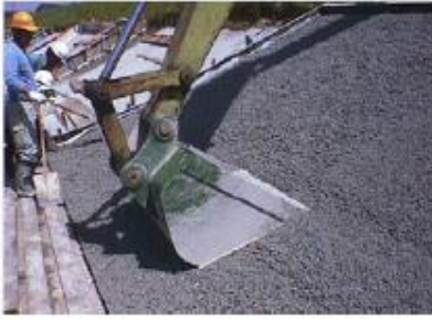
Photo-2 Compaction of revetment by a backhoe
