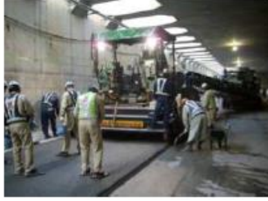
Photo-3 Spreading by an asphalt finisher
