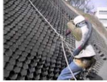
Photo-4 Slope protection by spraying (semi-dry)
