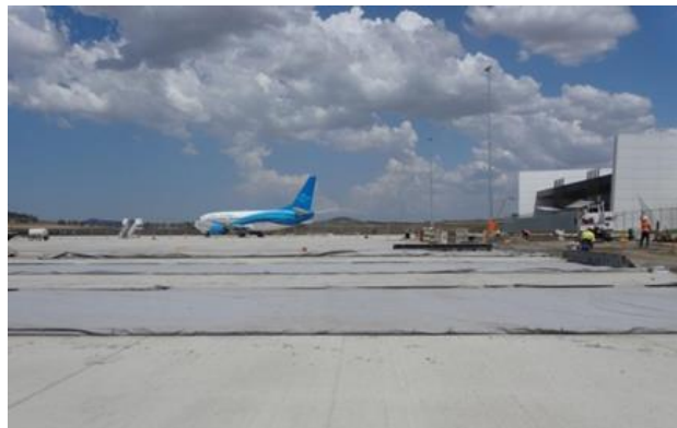
Image 6 - On site condition after construction.
