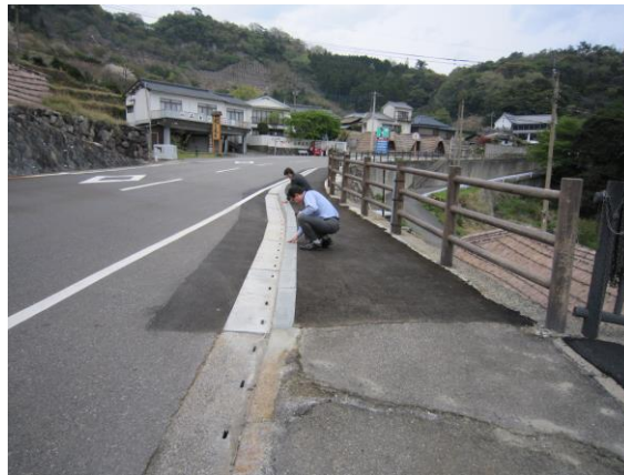
Image 4 - On site condition after construction.
