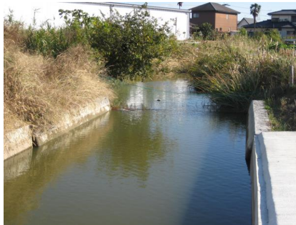
Image 2 - On site condition after 7 years from construction.
