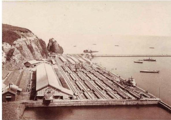
**Photograph 2: Construction of north breakwater (from Otaru Museum collection)**
