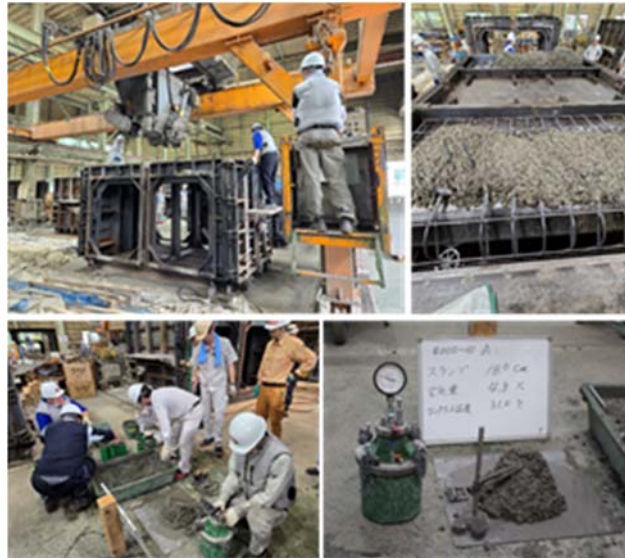
Photograph 1. Various tests and pouring into L-shaped retaining wall formwork
