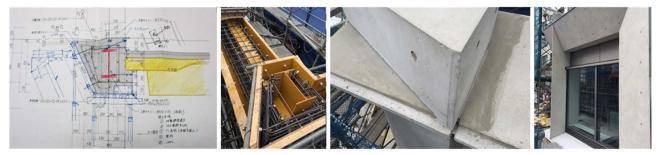
Fig. 11 Slender SRC column site casting
