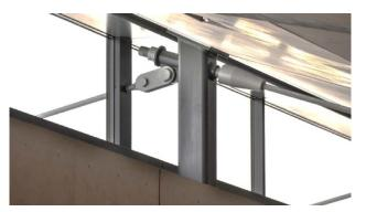
Fig. 8 Photo of cable fixing detail
