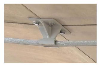
Fig. 11 Photo of precast panel fixing detail
