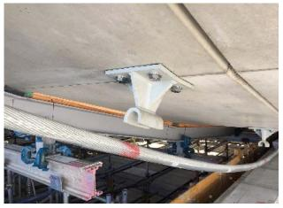
Fig. 12 Unstressed cable before tensioning work
