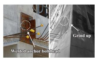
Fig. 11 Step 3: Base plate after welding is ground up
