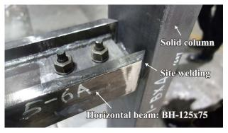
Fig. 7 Horizontal beam joint
