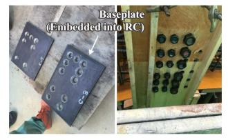
Fig. 10 Step 2: Base plate embedded in RC column
