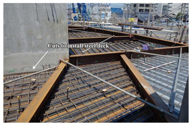
Fig. 13 Step-5: Installation of the steel beam and deck plate
