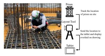
Fig. 9 Marking work on site
