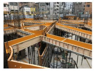
Fig. 7 Curved formwork and rebar layout
