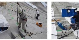
mortarInstalling (left) and tensioning (right) the prestressing cablesFig. 10Photographs from the PCaPC work phase
