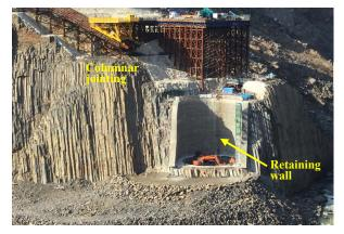
Fig. 4 Earth-retaining structure for PR2
