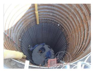
Fig. 5 Rebar assembly of foundation
