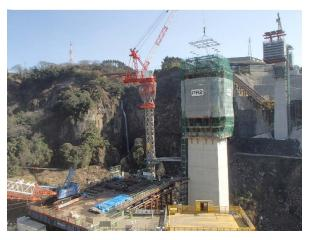
Fig. 6 Pier construction with a self-climbing system
