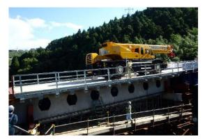
Fig. 4 Prototype non-metallic bridge
