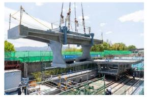
Fig. 7 Segment erection
