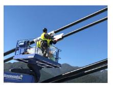
Fig. 5 Installation of the fire protection layer
