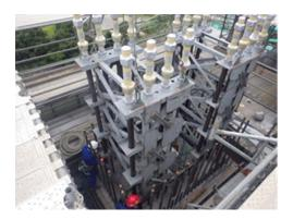
Fig. 7 Steel-concrete connection element made of steel frame in a pylon
