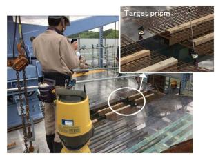
Fig. 6 Formwork setting by TS
