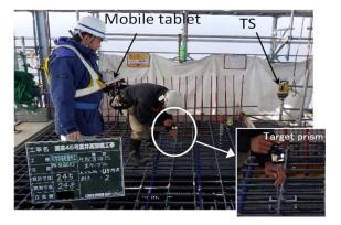
Fig. 8 PC steel tendon placement inspection
