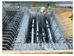
Fig. 5 Assembly inside a pier cap segment
