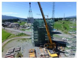
Fig. 4 Erection of a pier cap segment
