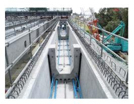
Fig. 8 Simplification of precast girder
