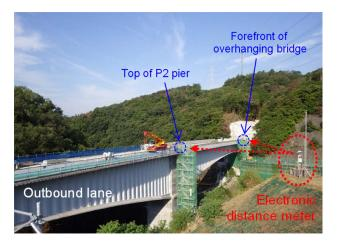
Fig. 8 Measurement of superstructure elevation
