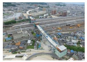
Fig. 6 In-progress construction at maximum cantilever length
