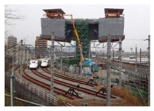
Fig. 7 Cantilever construction over the depot
