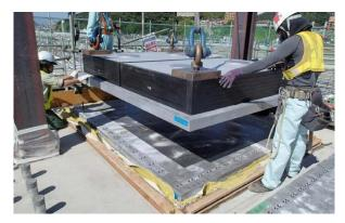
Fig. 5 On-site assembly of rubber bearings
