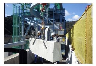
Fig. 8 Removal of existing bridge barrier
