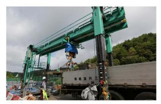
Fig. 8 Removal of existing slabs (phase I)
