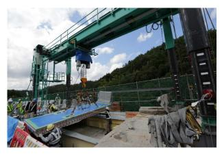
Fig. 9 Construction of PC slabs (phase II)
