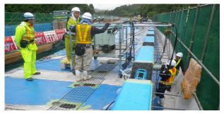
Fig. 10 Introducing the second tensioning (phase II)
