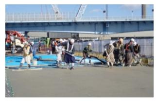
Fig. 9 Cast-in-place concrete deck slab
