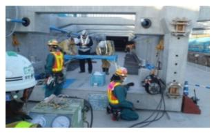
Fig. 6 External PC tendons tensioning (lower side)
