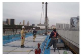
Fig. 8 Laying of PC panels
