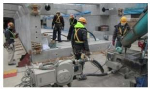
Fig. 7 Backfilling mortar into the gap under the bottom slab and levelling concrete
