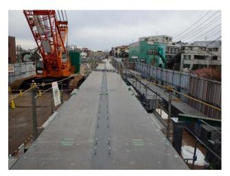
Fig. 6 Unification of the two main girders
