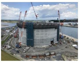
Fig. 9 Construction by the precast method
