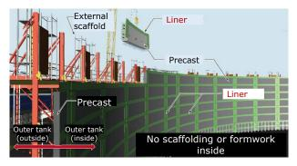
Fig. 3 Securing workspaces for machinery work
