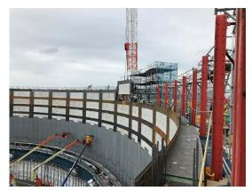
Fig. 10 Separate construction: civil and machinery, inside and outside outer tank
