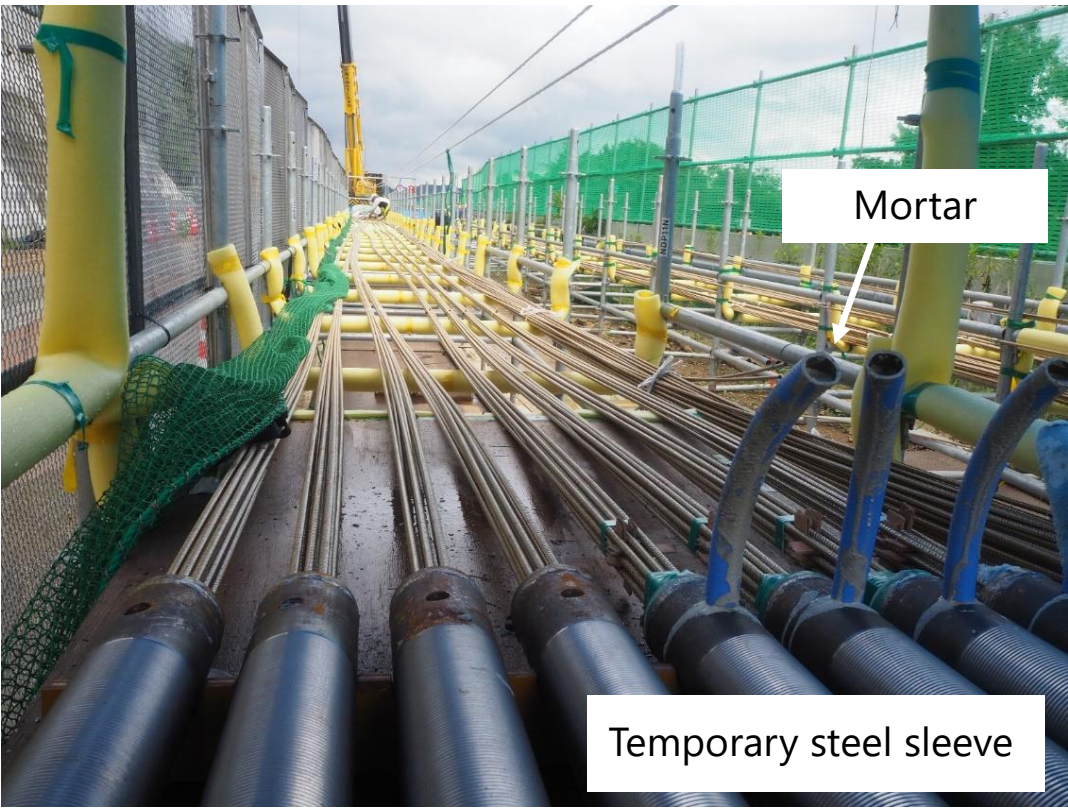
Deployment of aramid FRP rods for outer cables
