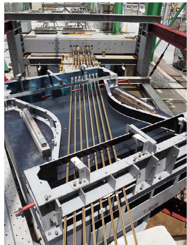
Aramid FRP rod placement (Butterfly Web)
