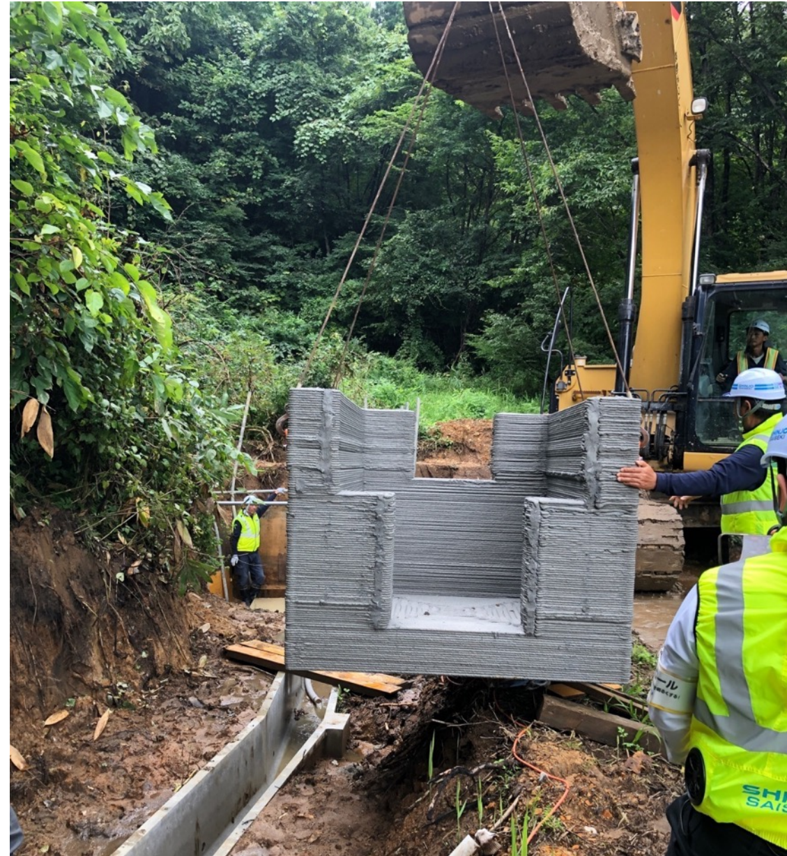
Standardized precast U-shaped gutters are used for the channels, but catch basins need to be customized to fit the local terrain, making 3D printing advantageous. 2022 October
