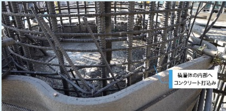
Rebar installation and concrete casting at construction site
