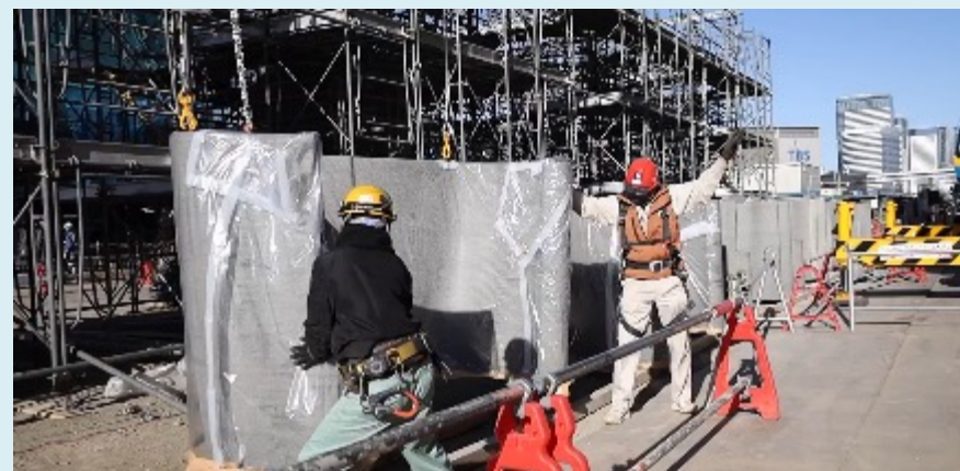
Transport and assemble the formwork the day after 3D printing
